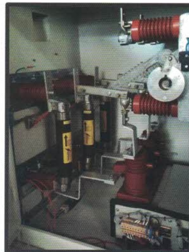
Figure 2: Sectional view of "TranSwitch"
